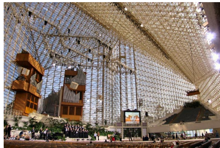
The Crystal Cathedral is a Protestant, Christian megachurch in Orange County, California. World-famous architect Philip Johnson designed the main sanctuary building, which was constructed using over 10,000 rectangular panes of glass and which can hold over 3,000 worshippers. When addressing issues such as faith and democracy, candidates running for office can reach anywhere from 20 worshippers in a small-town colonial church or thousands using these modern preaching mega-structures.
