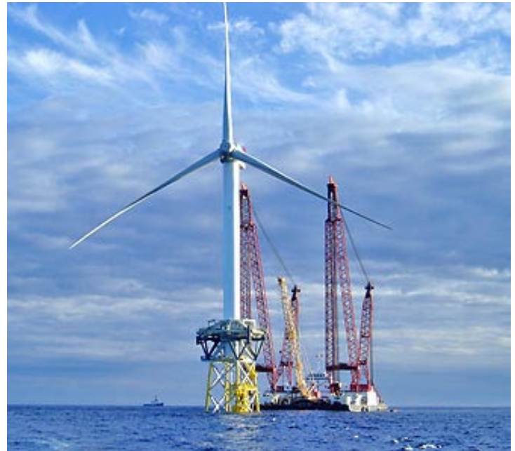
The world's largest wind turbine generator is currently undergoing testing in the North Sea off the East coast of Scotland. Each turbine weighs over 900 tons including the 360 foot tall tower which has to be anchored in deep water. It has an output of five Megawatts with each turbine blade being over 180 feet long.
